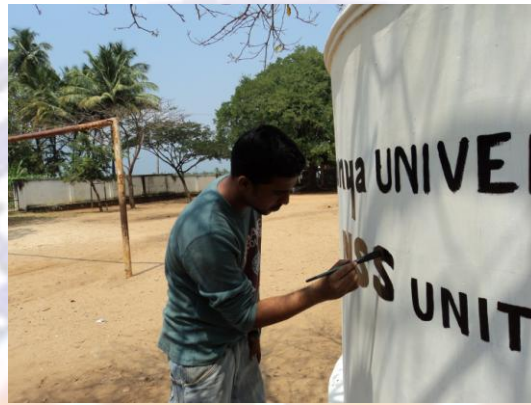
White washing Mathuvarayapuram school water tank
