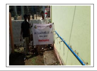
The plumbing works in the school campus was carried out in the afternoon session. The pipelines without proper pipe connections and the pipelines that were unfinished were repaired and new PVC pipes extra taps were provided for the school students to wash their plates during lunch. The pipelines were again checked for leakage and the mistakes were rectified. With this the second day of the camp came to an end.
